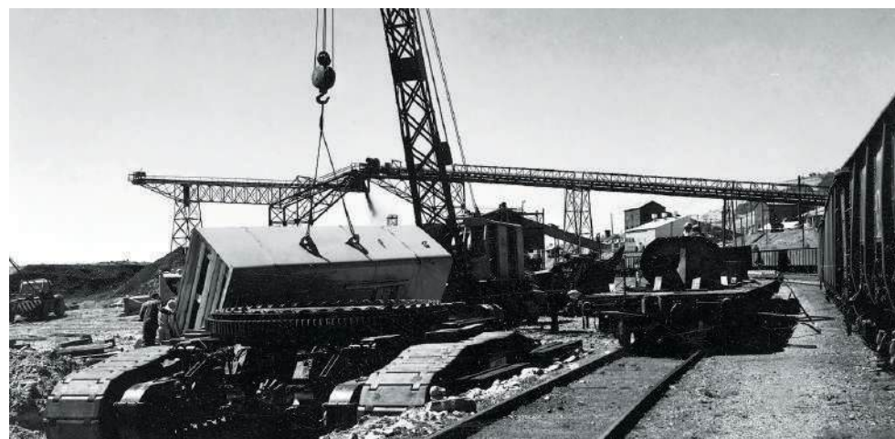
Construction of a rail access to transport iron ore, in 1950s, photo Special Collections SUU.
