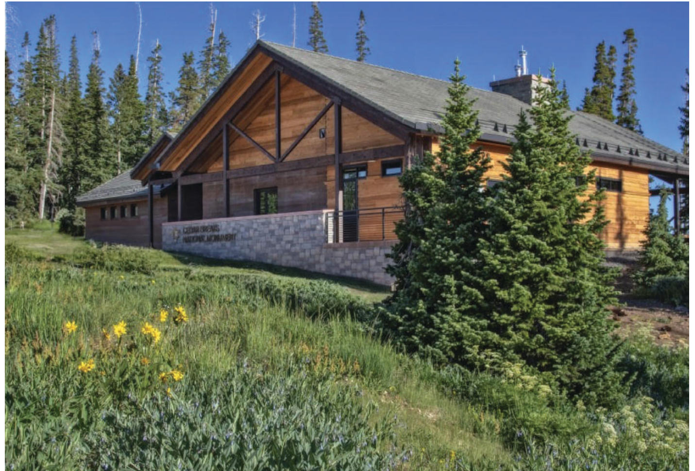
The new Cedar Breaks Visitor Contact Station. Zion National Park Forever Project Image / Wade Wixom
