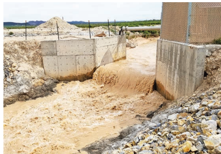
FLASH FLOOD WATERS WILL BE RE-CHANNELLED INTO A "LAZY RIVER" allowing the dirt and debris in the water to settle before being pumped into the recharge basin.
