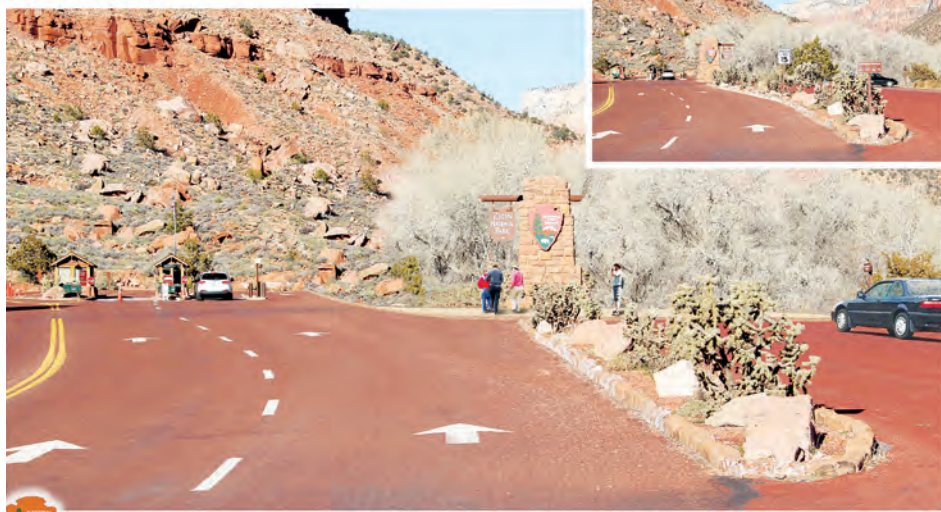
ENTRY MONUMENT RELOCATION ZION NATIONAL PARK 04/13/2014 COURTESY IMAGE
